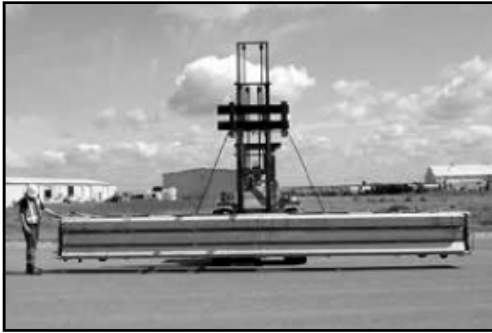
Figure 2. Use a crane, tractor or forklift to move the sections from the transport vehicle or trailer onto the job site.
