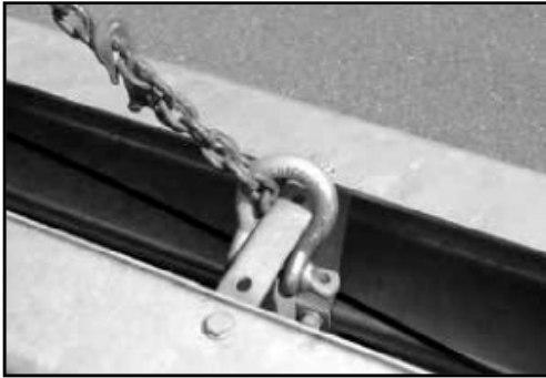
Figure 1. Use the holes located in the tops of the inboard diaphragms as two lifting points. Lift with a hook or clevis and a suitable cable or chain. Follow OSHA guidelines for safe forklift operation.
