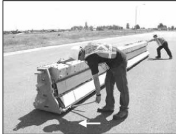
Figure 6. (QUICK TIP) If a section is difficult to get started moving, use the Hinge Pin as a lever to start the section moving.
