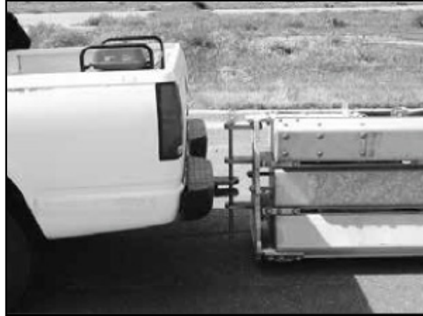
Figure 16. Attach the length of link barrier to a truck using a chain or a hinge pin as show above.
