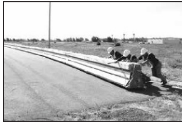
Figure 13: To deploy a barrier wall that is stored against a curb, move the end of the barrier out so that the truck can gain access.
