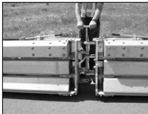
Figure 8. When all of the holes of the two section hinges are aligned, install the hinge pin. The pin must be fully installed.
