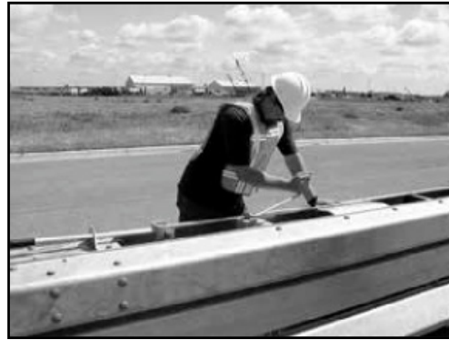
Figure 3. Manually jacking a section
