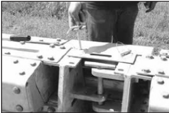
Figure 11: Rotate the cover up to the closed position and install the two keeper pins through the top as shown below.
