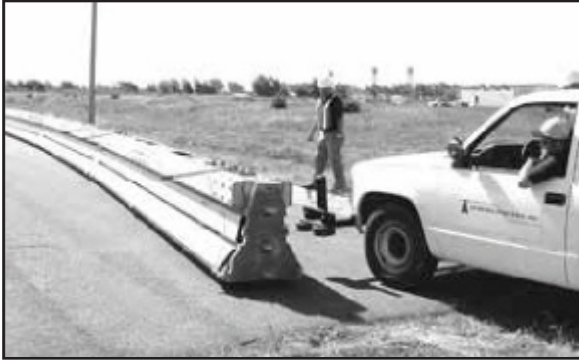
Figure 14: Push the barrier over with the vehicle as you drive along the side of the barrier. The tiller handles must be pointed in the direction of desired movement.
