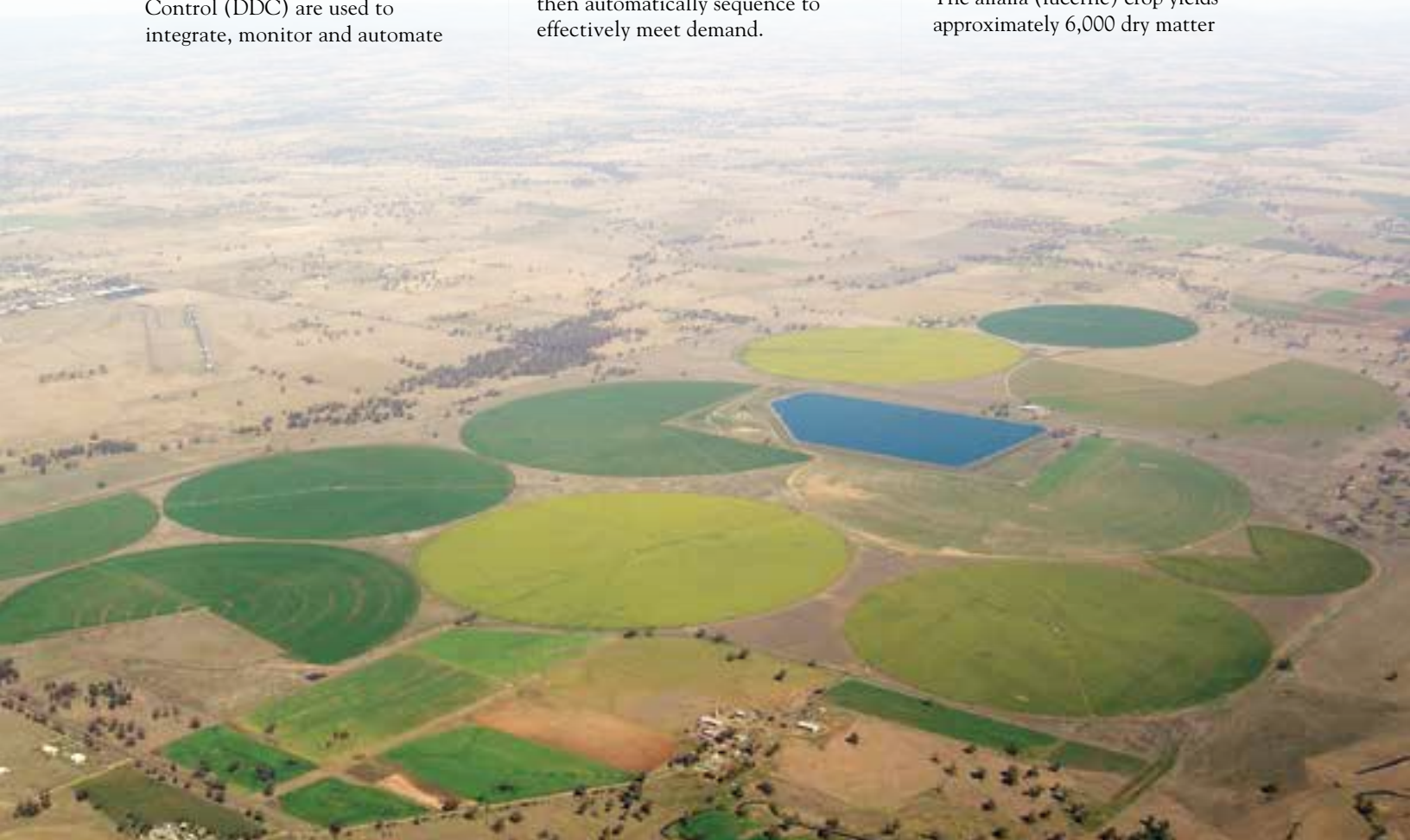
Aerial view of the Tamworth City wastewater reuse project in Australia. The wastewater storage pond can hold up to 396 million gallons (1,500 ML) of water, which is then pumped onto local crops through 13 new Zimmatic center pivots.
