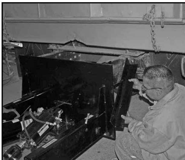
Figure 7. Install side Channel Braces.
