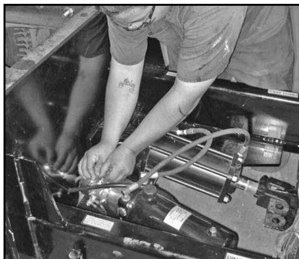
Figure 14. Attached to Support Structure.
