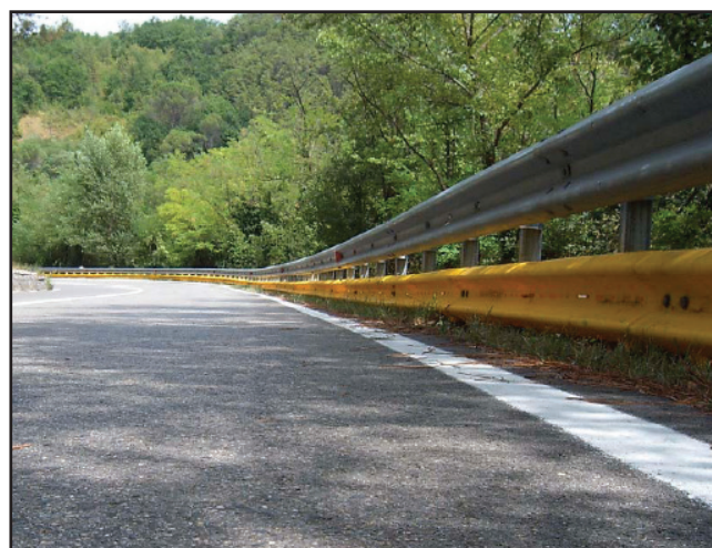
Figure 9 - Leveling and final fixing of the protection
