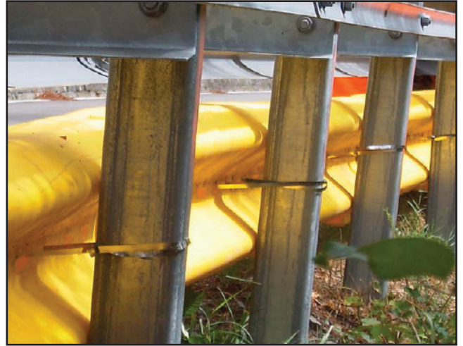
Figure 4 - Fixing caps using clamps
