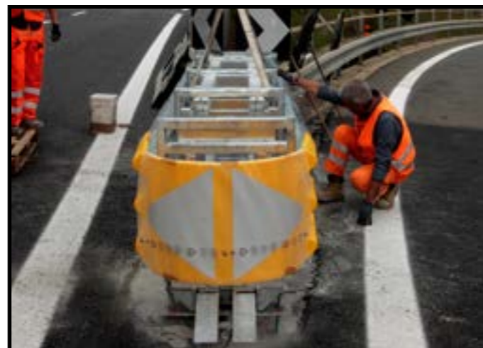
Figure 1c) TAU Tube™ placing
