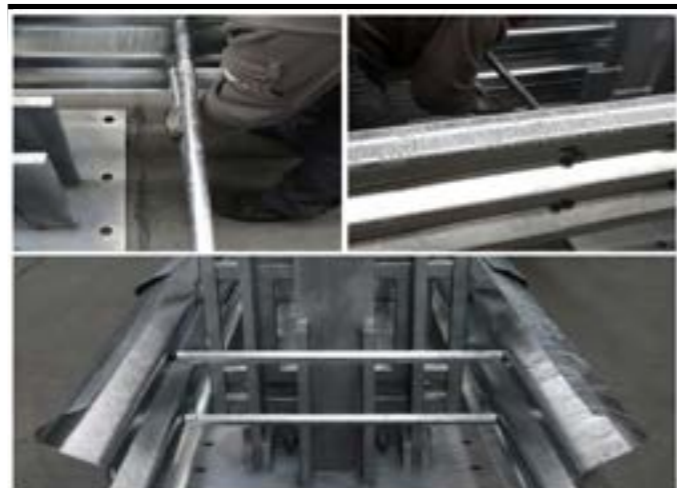
Figure 12 Mounting of the tube crosspieces
