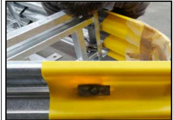
Figure 11a Fixing the nose to the panels
