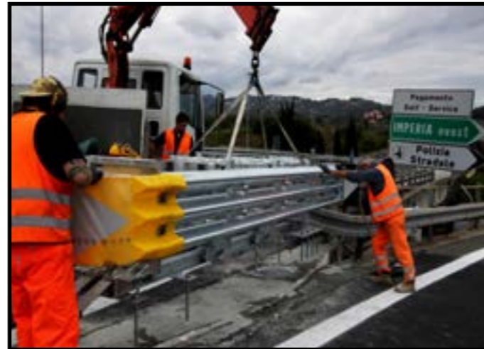
Figure 1b) TAU Tube™ placing
