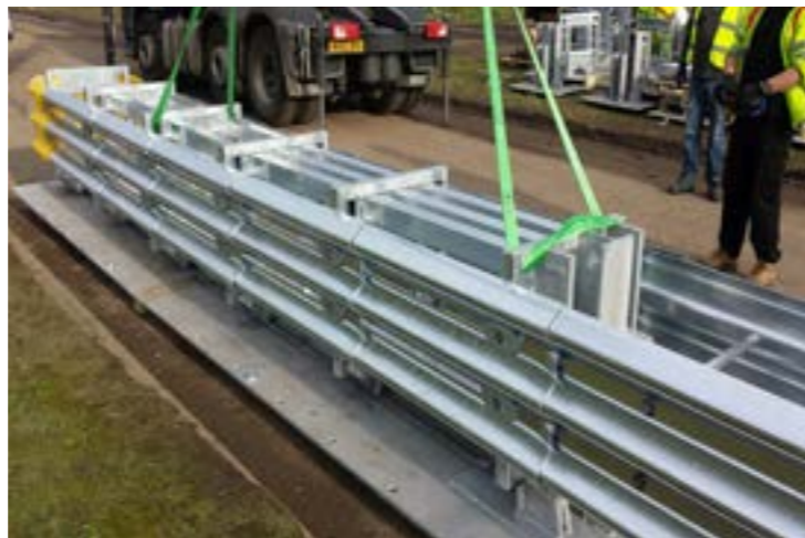
Figure 15 Positioning Tau Tube® pre-assembled on plate
