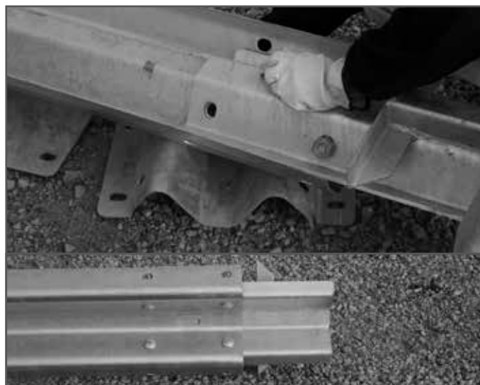
Attach Slider Bracket to Rail 2.
