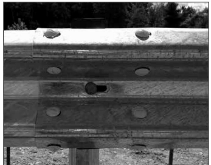
Shear Bolts at Rail 3 and 4 Connection
