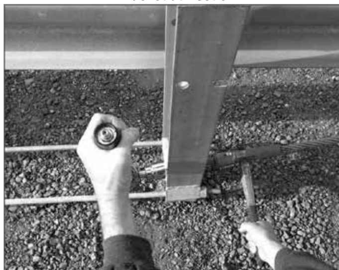
Torque cable nut to 60 ft.-lb. at Post 2
