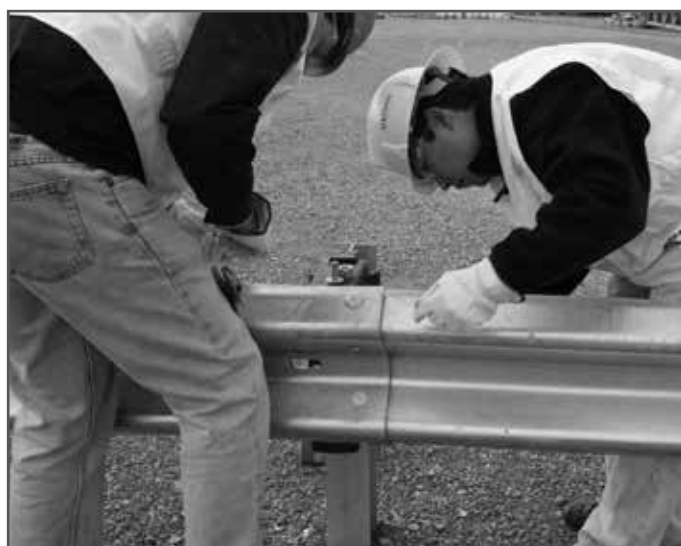
Shear Bolts at Rail 2 and Connection
