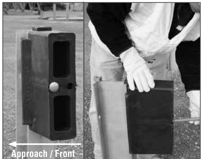
Install Blockout at Post 5
