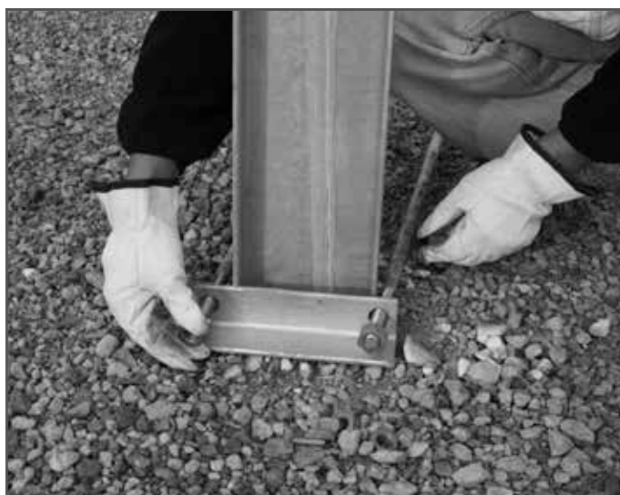
Ground Strut Tension Rods Attached at Post 1
