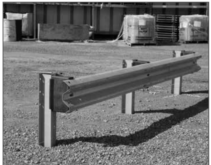
Existing Trailing / Back Guardrail
