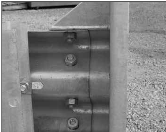
Impact Head Installed
