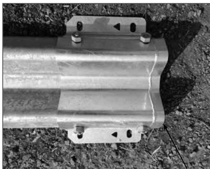
Attach Slider Panel (Front) to Rail 1.
