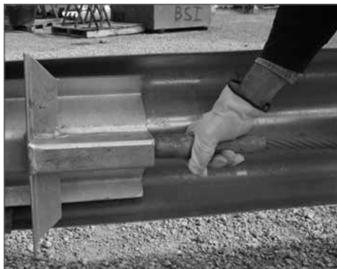
Install Trailing / Back End of Cable Through Bracket at Post 3
